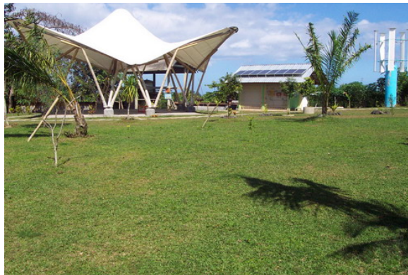
After transformation to the outdoor park section of the educational center. The bamboo building still without its tarpaulin roof
