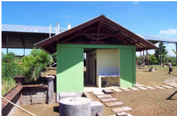
The new toilet block with the methane producing biodigester in front (mostly under ground). The new large scale composting facility can be seen in the background
