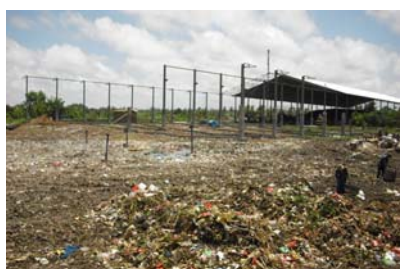
Phase 2 expansion to 2400 m 2 Sep. 2009 (for total 60 tons/day)
