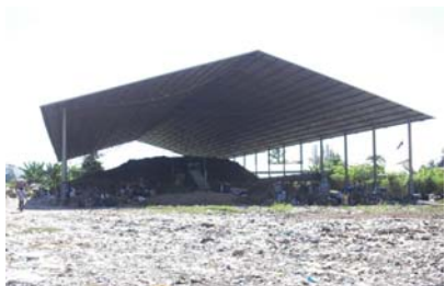
Phase 1 composting building of 2400 m 2 (30 tons/day)
