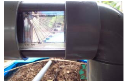
Flow meters, self-made to save cost
