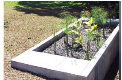
Wastewater Garden for cleaning effluent from biogas rector
