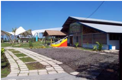
After restoring the old landfill for the environmental park
